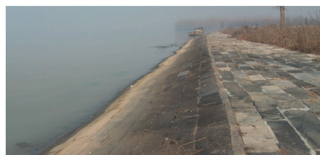
The dam at Hongze Lake is, with regard to canal technology, one of the canal's most important historic sites.
